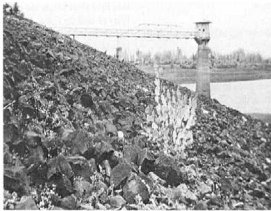
Figure 6-46.—Riprap on upstream slope of an earthfill dam. Dam is in excellent condition after 50 years of service. The structure is Cold Springs Dam, which forms an offstream reservoir on the Umatilla Project in Oregon. IO-2194.
